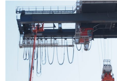
Crane Condition Survey
